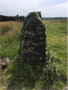
A dry stone wall in section, showing the way it was constructed A weir, which was constructed to provide water power
