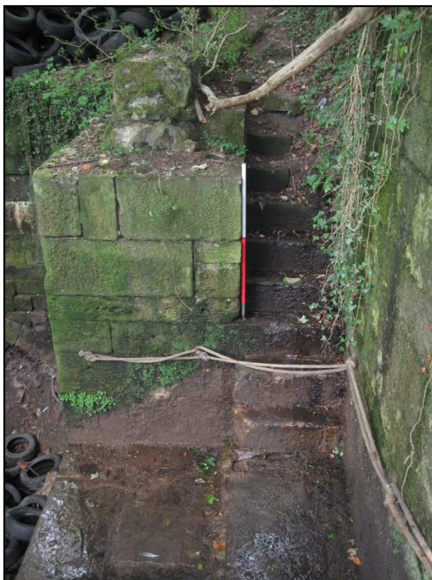
Figure 19: Looking west. Shot of steps on northern axle bed.
