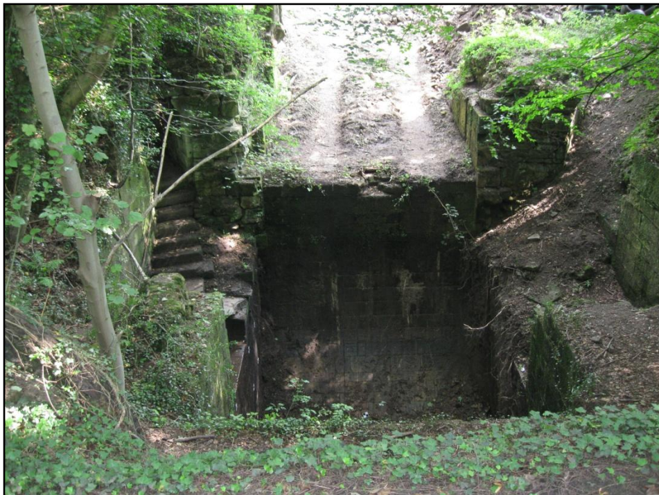
Figure 21: View from above wheel pit. Looking east.
