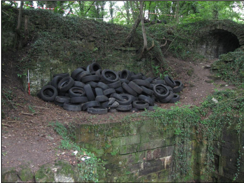
Figure 22 – View from south side axle bed. Top of east facing section visible.
