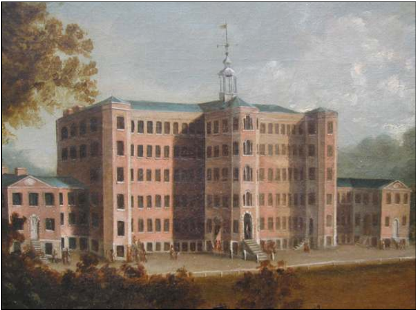
Figure 9: Artist impression (Francis Jukes) of the southeast facing façade of Mellor Mill c.1803, showing stone built ground floor and red brick superstructure
