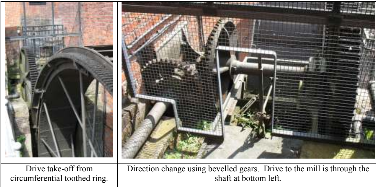
Figure 2: Example of power take off from waterwheel using a geared ring and bevel gears. Picture taken at Portland Basin, Ashton-under-Lyne.
