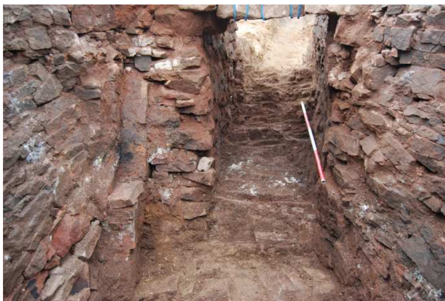
Figure 21. A view from inside the Pot looking through the Eye and along the flue.
